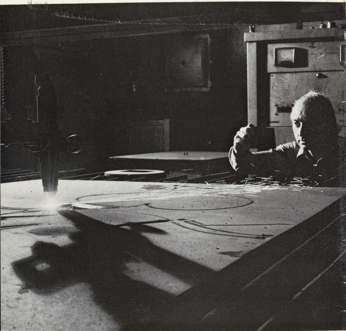
Ismond Rosen, plasma arc cutting at Plascut Ltd, Rotherham.
